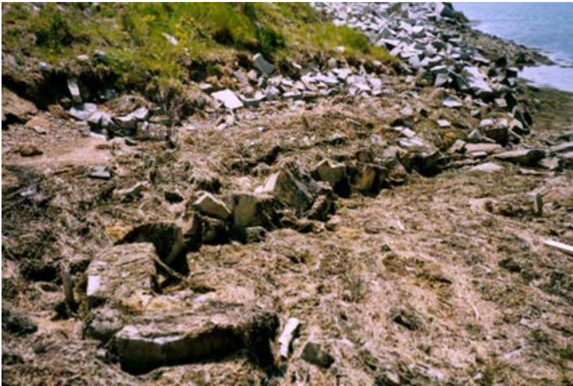
Figure 69: Wave attenuation barrier inserted in 1998 to slow the eroding effects of spring storms while the plantings took root. Granite detritus remains from the former quarrying industry can be seen in the upper half of the image, left at the site on purpose, to compare rates of plant colonization (Rahmani 1998).
